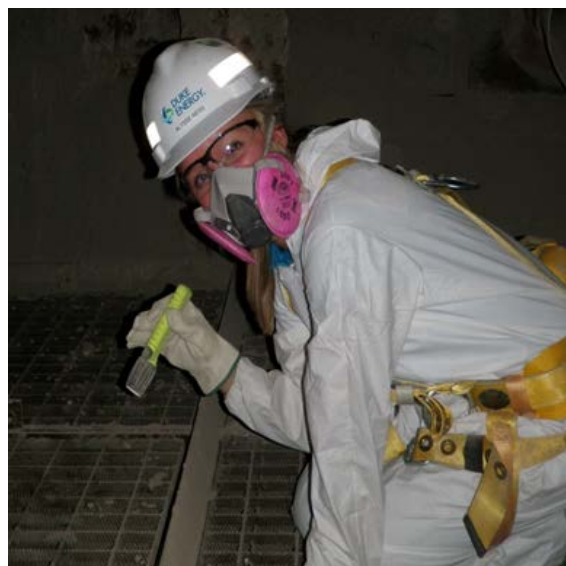
Alysse Ness inspecting selective catalytic reduction equipment, used to remove NO x from the flue gas airstream.
